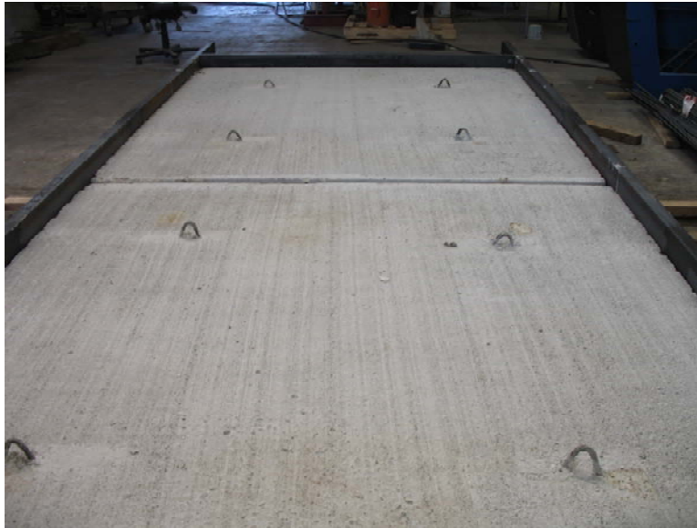
Figure 4-1: PCPs Prior to Casting CIP Slab
