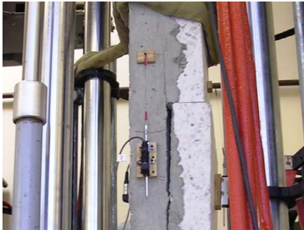
Figure 4-26: Delamination of PCPs during Tension Test
