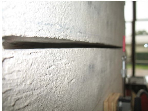
Figure 4-28: Saw-Cut of CIP
