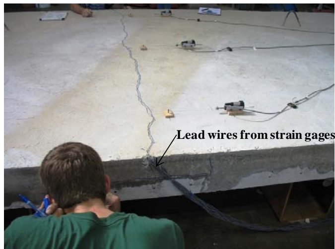
Figure 4-9: First Crack due to Lead Wires
