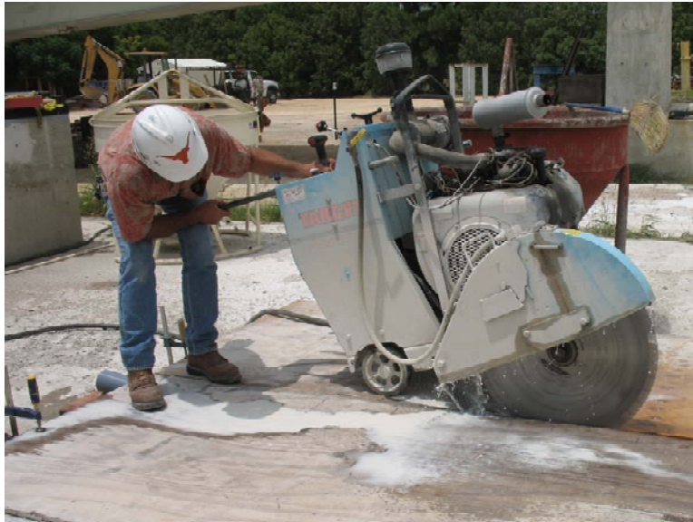
Figure 4-21: Concrete Saw used to Cut PCPs
