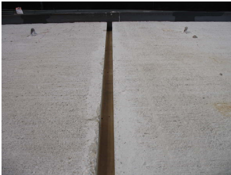
Figure 4-2: Gap between PCPs
