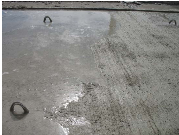
Figure 2-12: Beginning of Flooding PCPs for Curing
