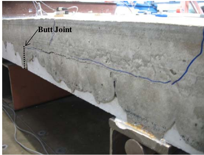
Figure 4-8: Delamination during Constant Bending Moment Test
